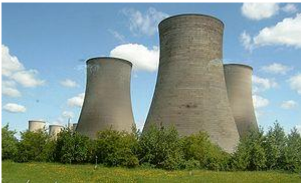
and the natural draft wet cooling hyperbolic towers at Didcot Power Station , UK show hyperbolic designs.
